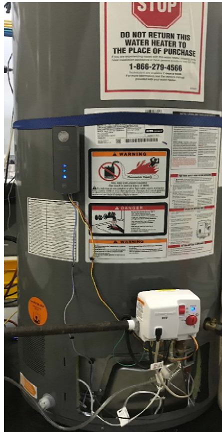
Figure 1. Rheem EcoNet WiFi Module
